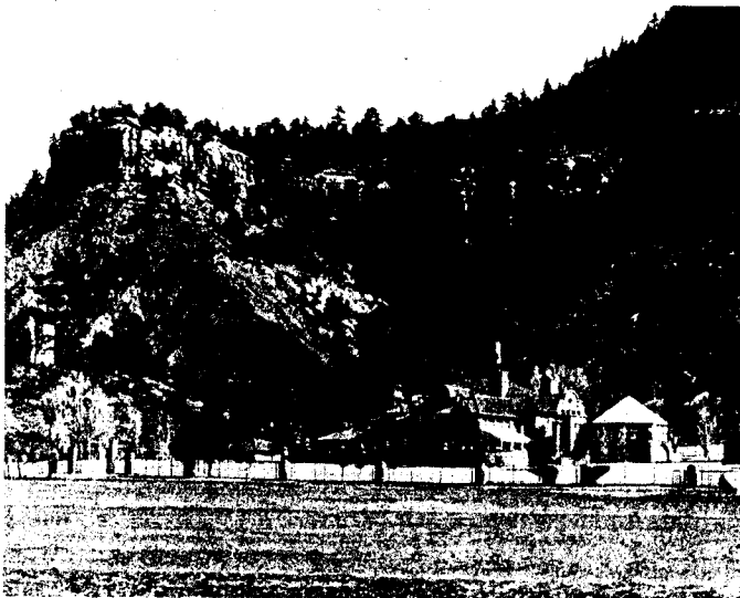
Figure 4. Casa Grande. Began for Bartlett in 1908.
