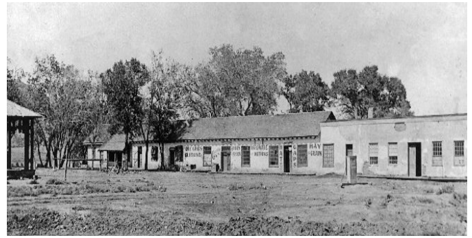
Cimarron News and Press . The Lail family has used it as a residence since 1908. The original adobe structure, severely damaged by fire in 1939, is mentioned in Zane Grey's book Fighting Caravans .
